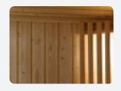
58 mm fir walls and ceiling reflect heat without added insulation and minimised use of materials
